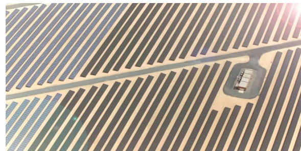
Masdar PV Plant
