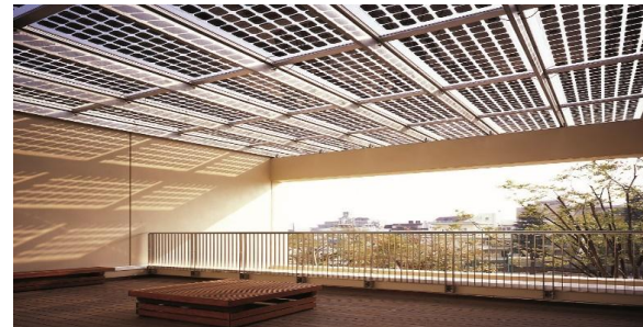
Tokyo Guanghua Primary School BIPV Project
