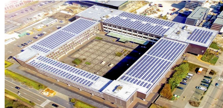
Genk City Hall Rooftop PV Project
