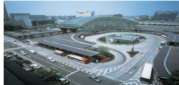
Kanazawa Bus Station BIPV Project
