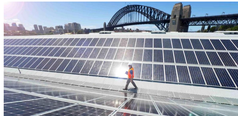
Sydney Opera House Rooftop PV Project
