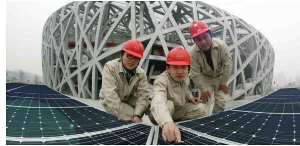
Beijing National Stadium BIPV Project
