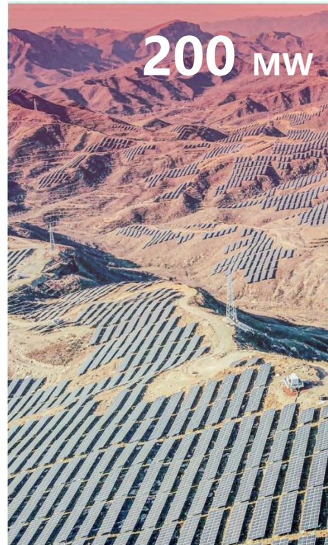
Shunping Rural PV Plant
